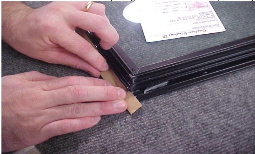
Any exposed gasket will be trimmed off later. The gasket should be lined up with the edge of the flange but not protrude out past the edge of the flange.
